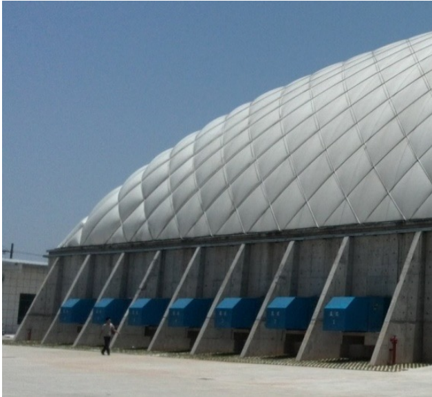
Direct-drive centrifugal blower
