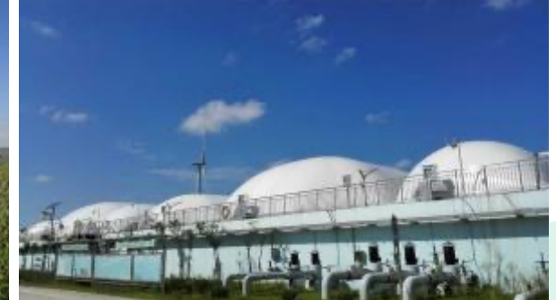
■ Sewage Treatment Plant
